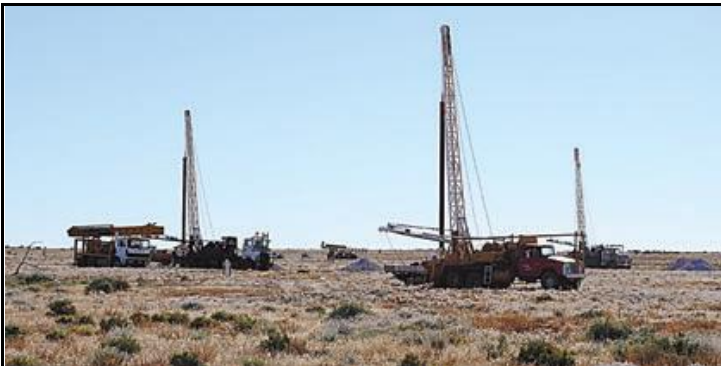
Currently there are 3 Caldwell drills, 3 investigator drills, 1 dozer, 2 Excavators and a dump truck working on 'Donna's Rush'
